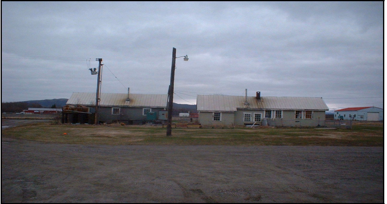
Photograph 1: Looking north at the CAA utility buildings (RUS-033 and RUS-034) that are eligible for the National Register of Historic Places.
