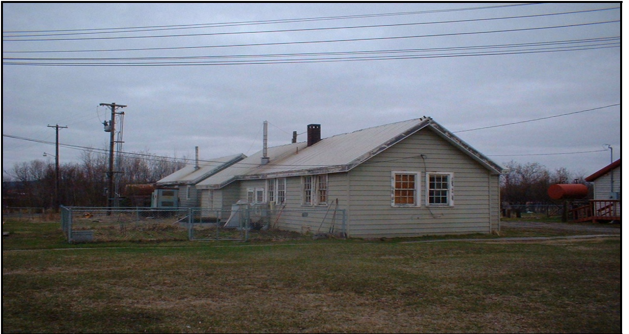
Photograph 2: Looking northwest at the CAA utility buildings (RUS-033 and RUS-034) that are eligible for the National Register of Historic Places.
